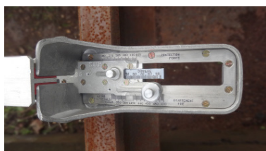
Control Track Guide between Guard-Rails and Width of Switch-Opening
